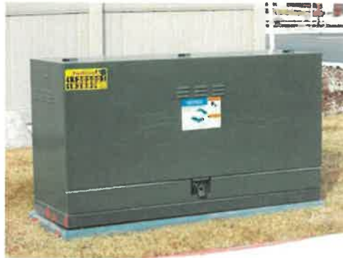
Figure 48—Three-Phase Sectionalizing Cabinet
