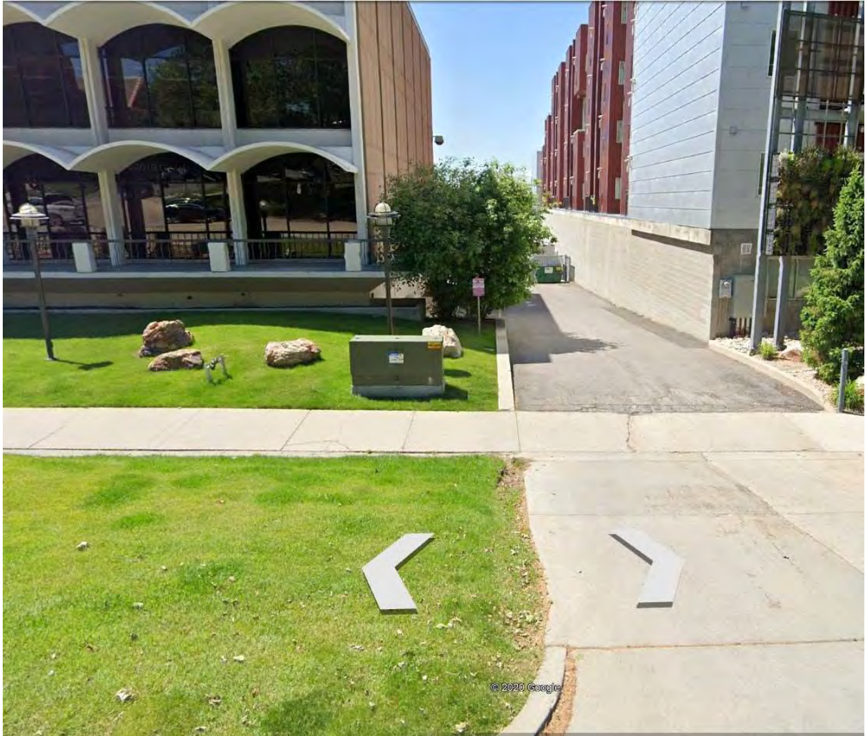
Existing Sectionalizer at 340 E. South Temple
