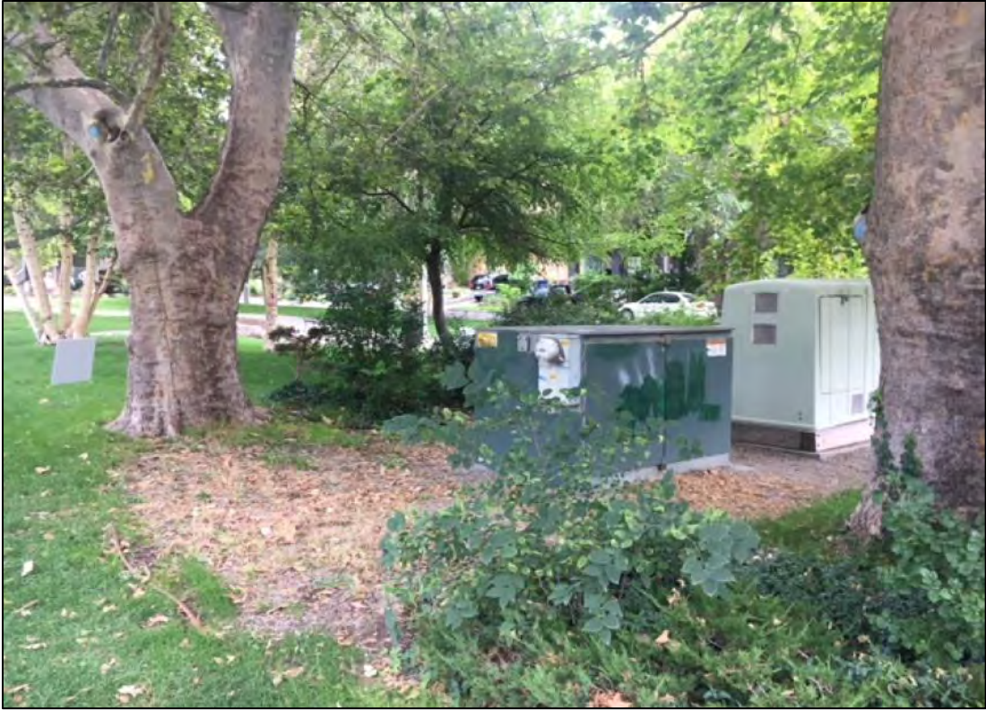
North/Eastern View of Existing Well
