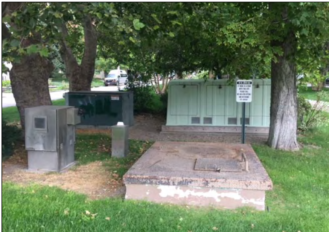
View of Existing Well
